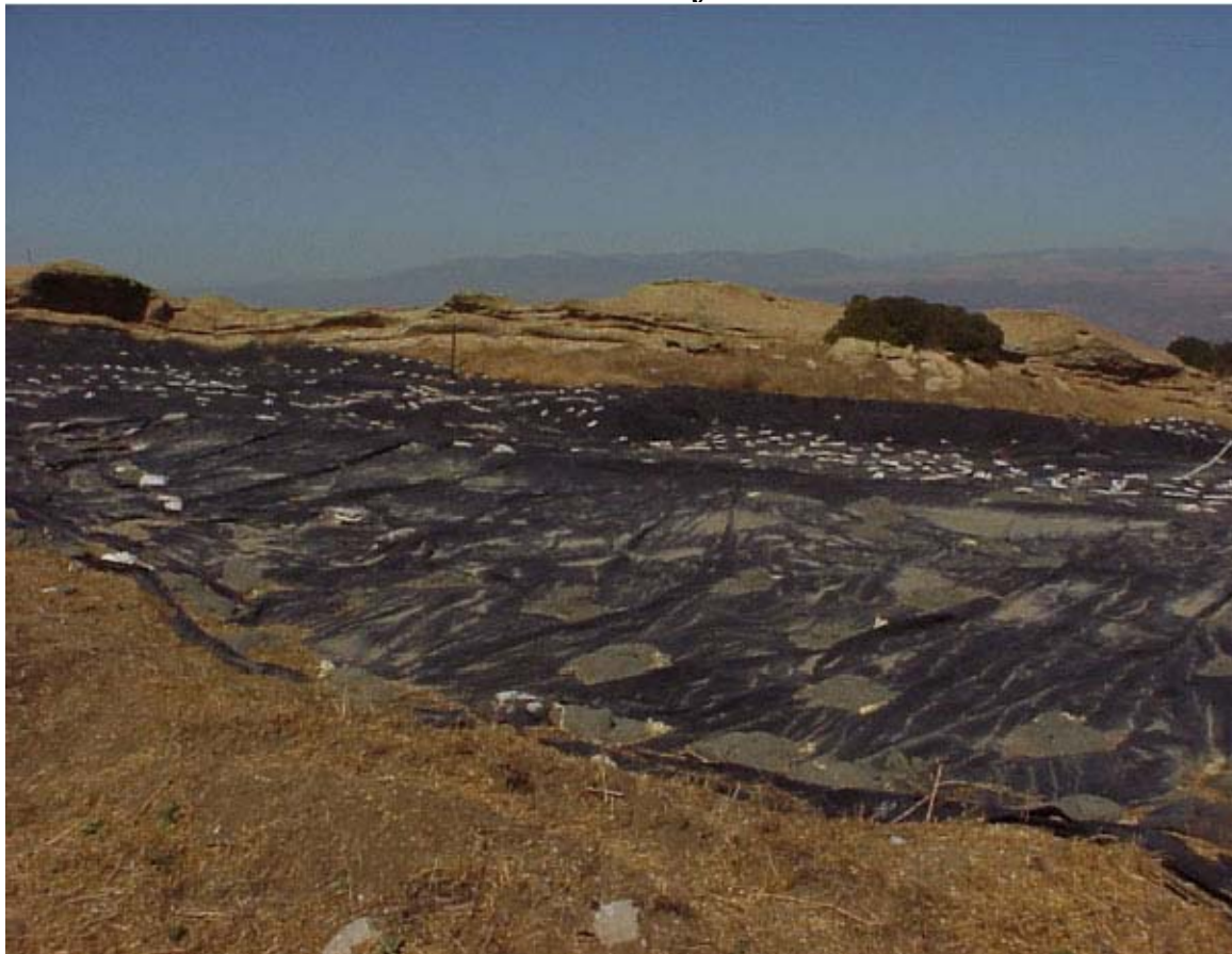
Figure 8. Site of former Sodium Disposal Facility. The view is looking northwest towards Brandeis-Bardin Institute and Simi Valley.
